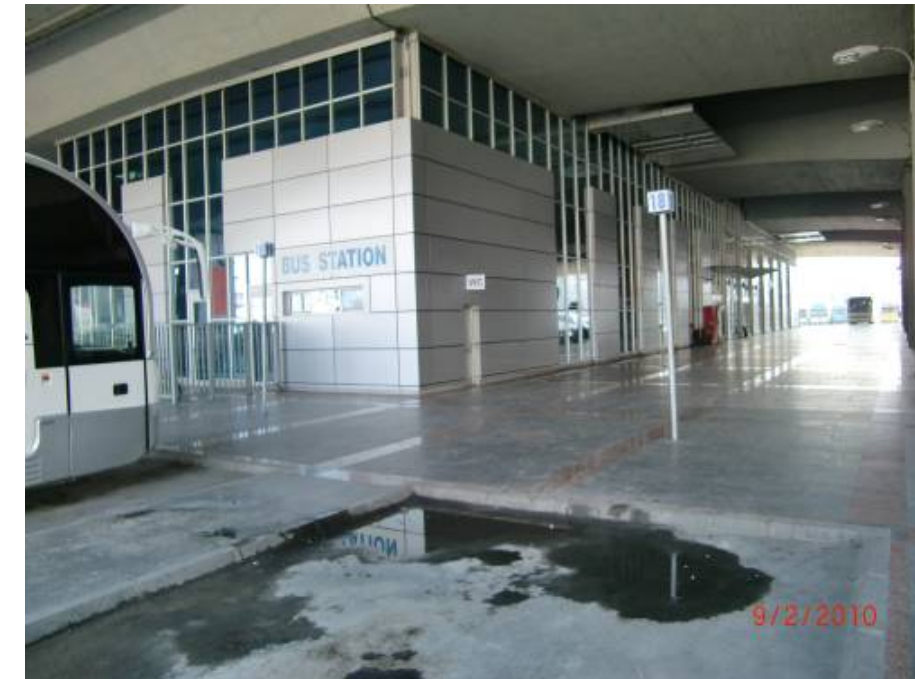
IMAGE 20, REGIONAL BUS STATION UNDERNEATH TRAIN PLATFORMS AT TRANSPORTEN CENTAR, SOURCE: IDOM
